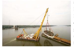
shaped horizontal section with 42\*14m) are so large that the possibility of lifting was doubt. Because of the limit of crane capacity the concrete elements are formwork of the concrete pier and not only protecting elements of the underwater site. So we didn't use steel elements but only concrete ones. The concrete shell
