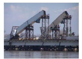
The most exciting, complicated and difficult task will be the shipping of the arch bridge. The contractor assembles the structure on the left bank of the river. After the completion of the arch structure they let down the scaffolding, thread and stress the cables lifting with that the superstructure from its supports. After that they build temporary stiffening
